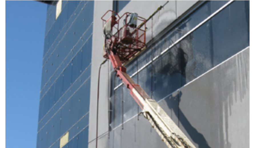
Figure 3: Field testing for resistance to water penetration
