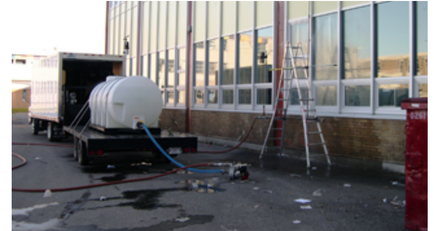
Figure 21: Portable water reservoir and pump system
