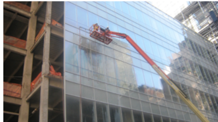
Figure 20: Calibrated sprinkler rack hung from motorized man lift
