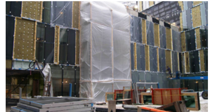
Figure 22: Temporary exterior heating via test specimen
