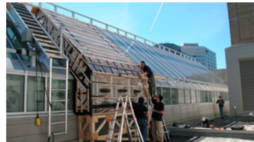
Figure 13: Exterior test chamber used to test a skylight section
