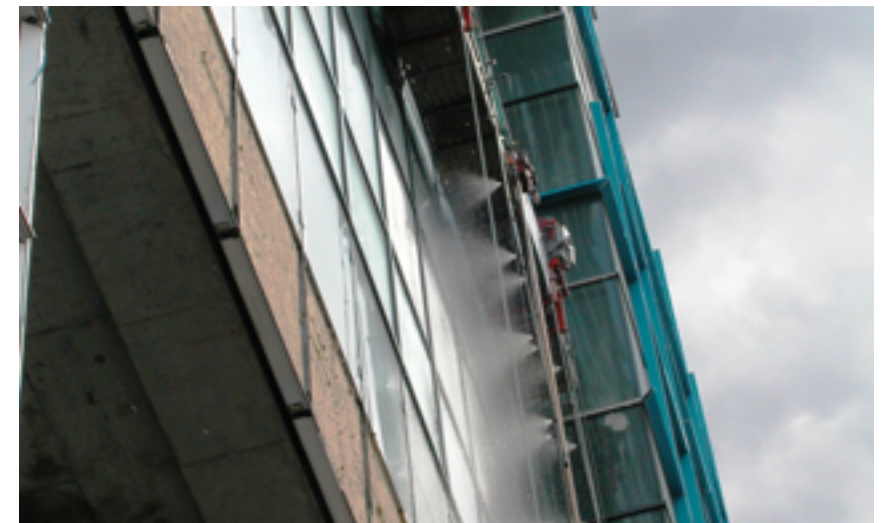
Figure 4: Field testing for resistance to water penetration
