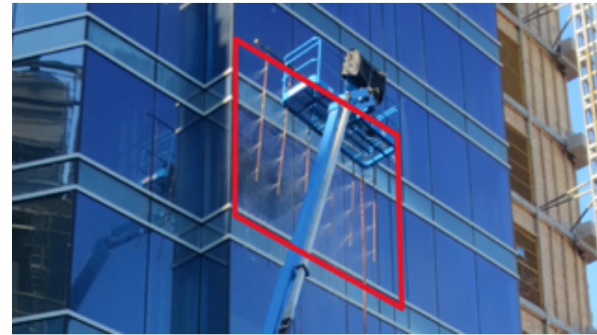
Figure 8: Identification of representative area for field testing (metal and glass curtain wall
